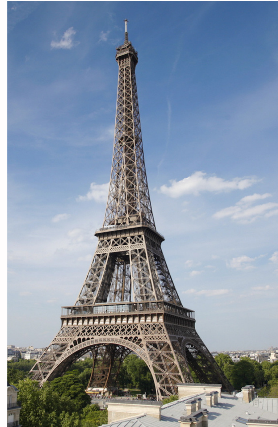
Eiffel Tower, Paris Gerda Guide Rails
