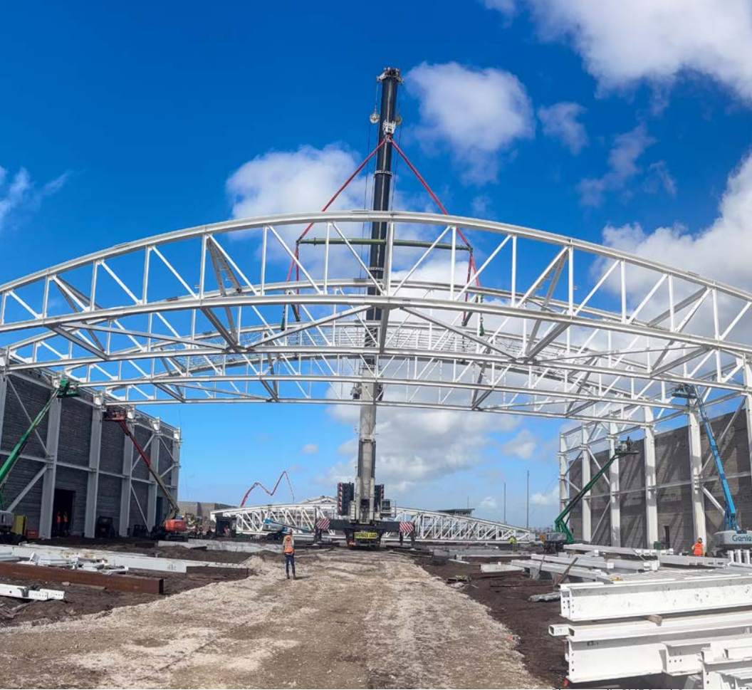
Photo credit GMF Steel Group
