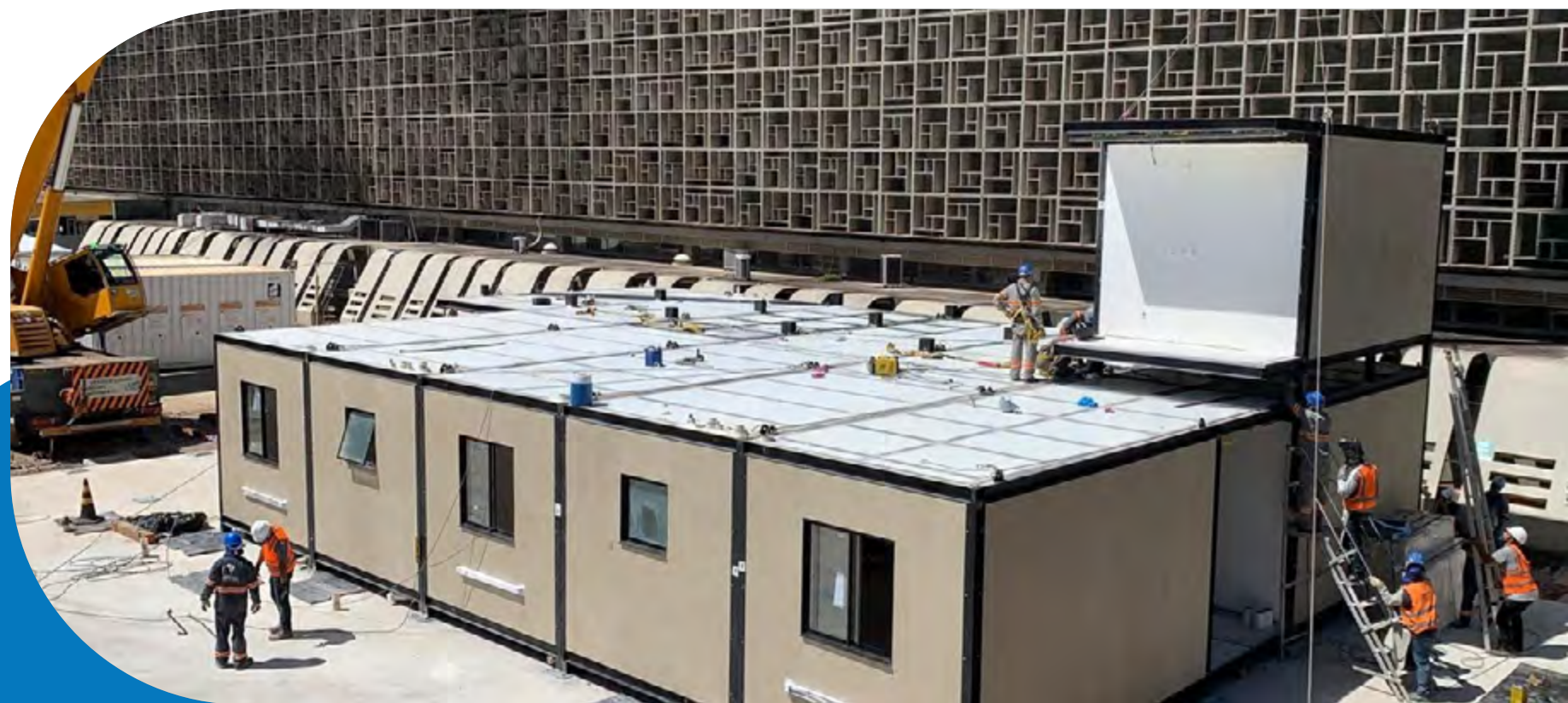
Brasil ao Cubo's modular construction technique uses steel as the main raw material.
