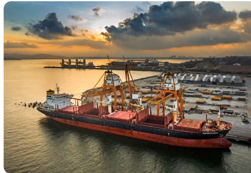
Port terminal, Vitória (ES)
