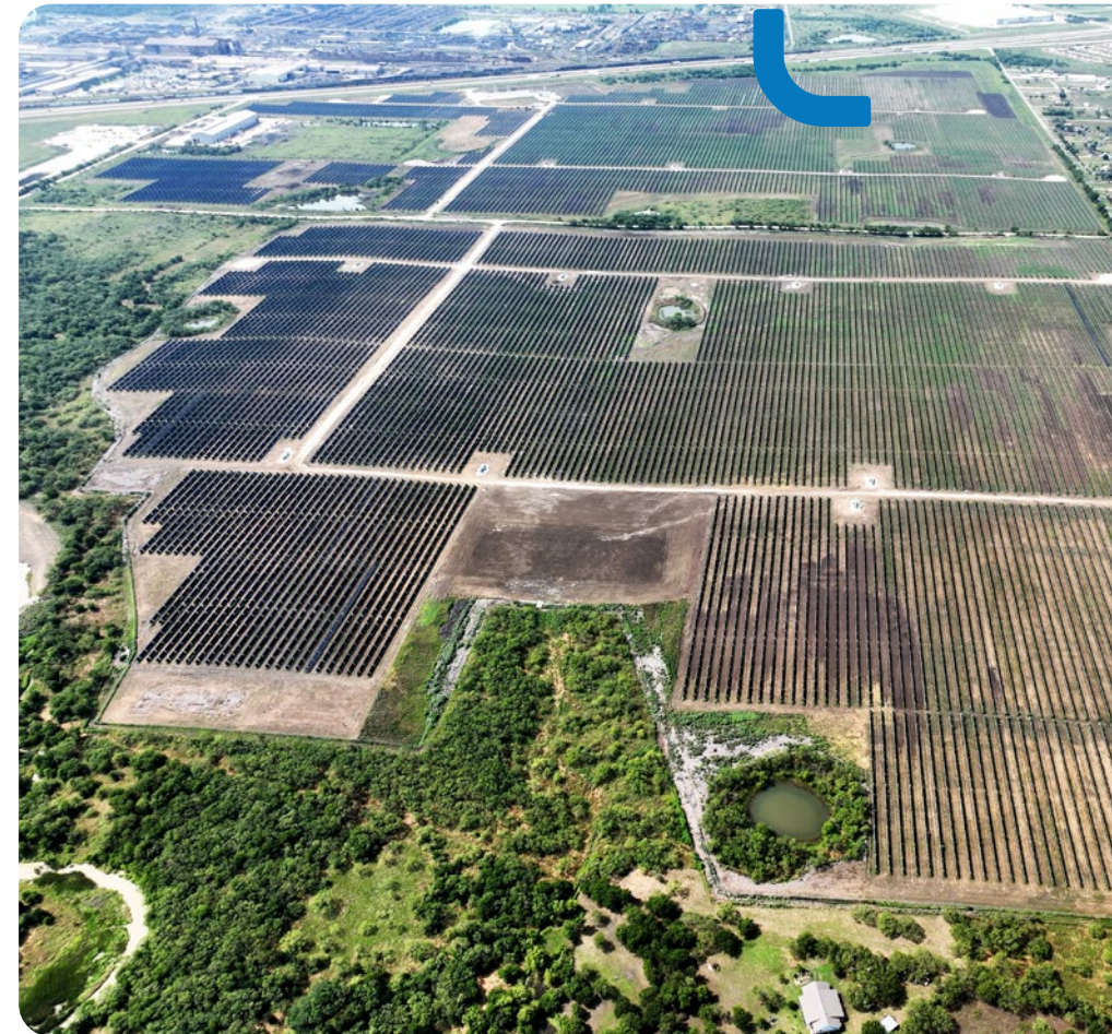
Midlothian solar farm, USA
